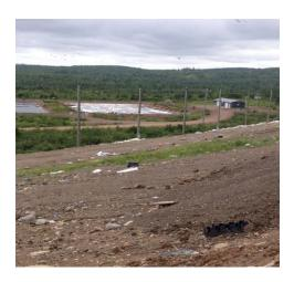
This is the only 2<sup>nd</sup> generation lined landfill with full leachate treatment centre in the Province. The system has liners in the ground which collects any leachate and directs it to a leachate treatment plant. The plant then treats the leachate before it is released to the environment. Leachate monitoring test is reported monthly.
